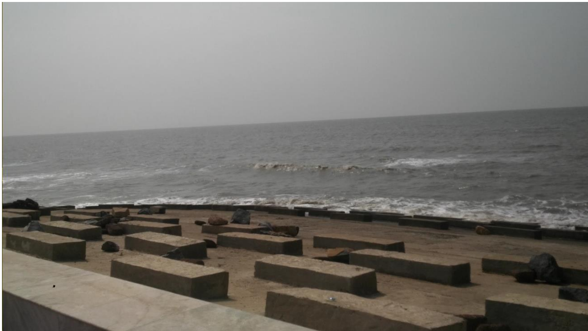
Photo 4.4.6 Another view of Friction Blocks
