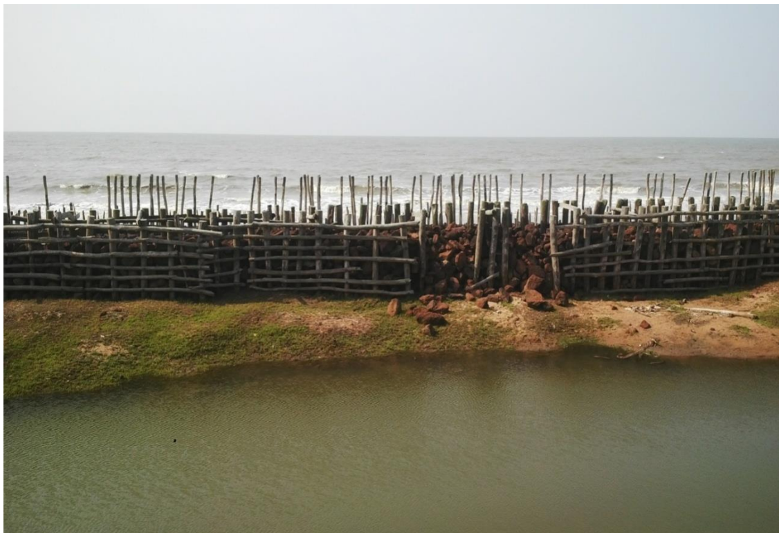
Photo 4.4.11 Seawall at Tajpur showing rubble fill between timber piles
