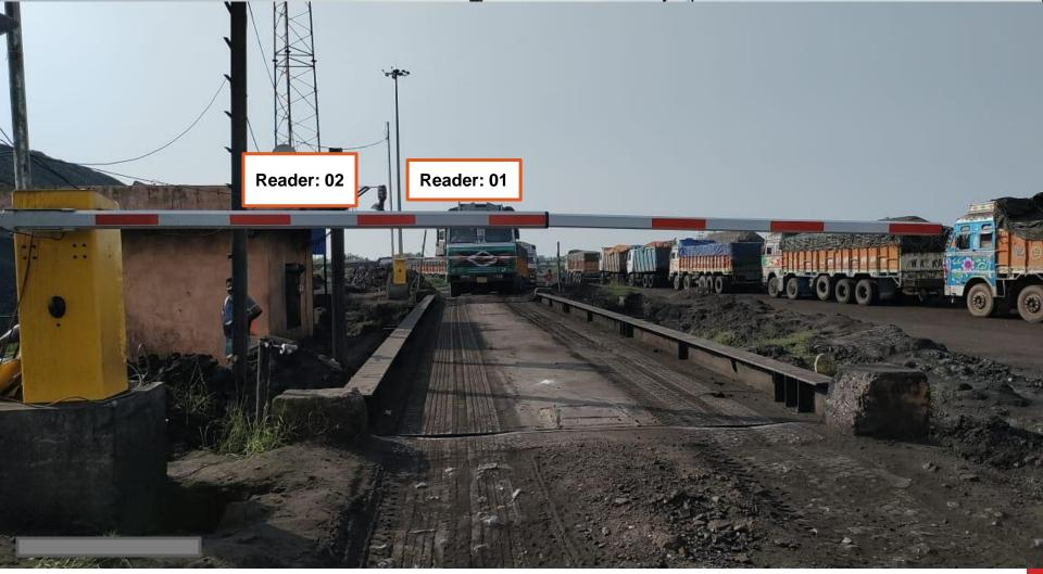
After successfully exit of the vehicle from weighbridge ramp Boom barrier (exit side) will close automatically.
