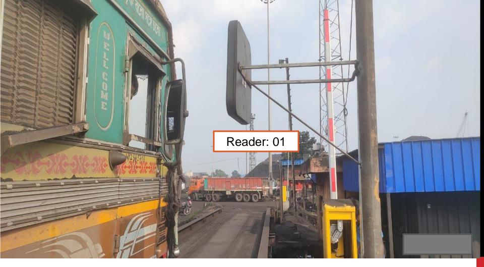
On flashing vehicle RFID card at RFID reader(01) the boom barrier at the entry side opens.
