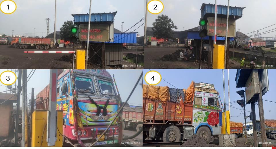
After successfully weighment (refer to Picture 1) of the vehicle Exit Boom Barrier will open automatically (refer to Picture 2) and Green Signal light indication for move out the vehicle form Weighbridge ramp (refer to Picture 3,4). LED display will show the vehicle number and weight (refer to Picture 2).
